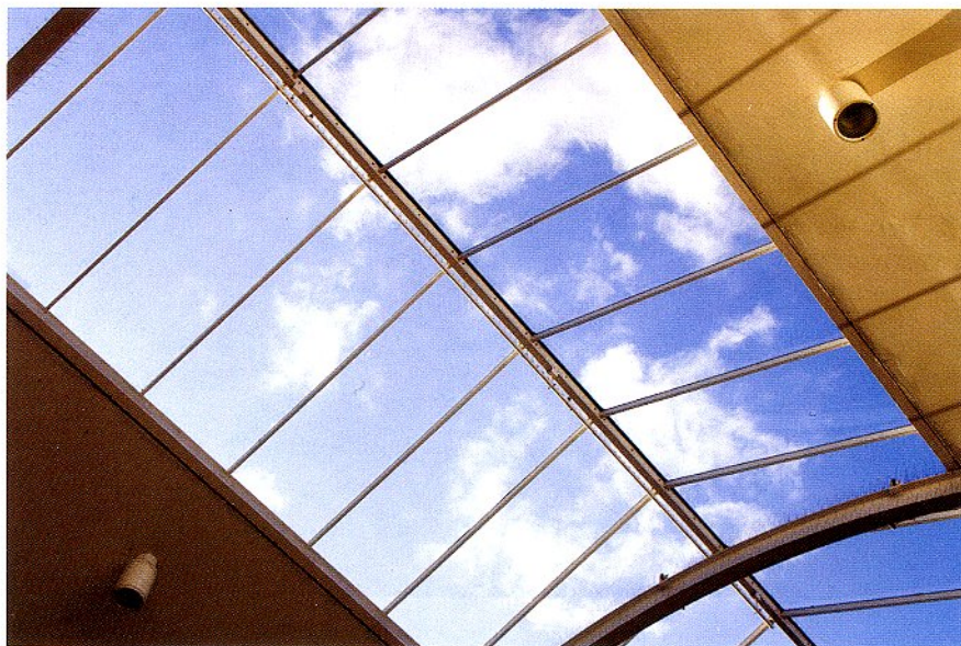
Using natural lighting to reduce energy use can help wineries save money while promoting sustainable practices.
